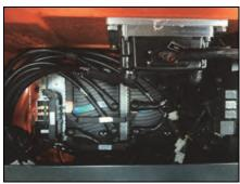
Clean the control panel with 205 kPa (30 psi) maximum air pressure, until dust is removed from the control panel.
